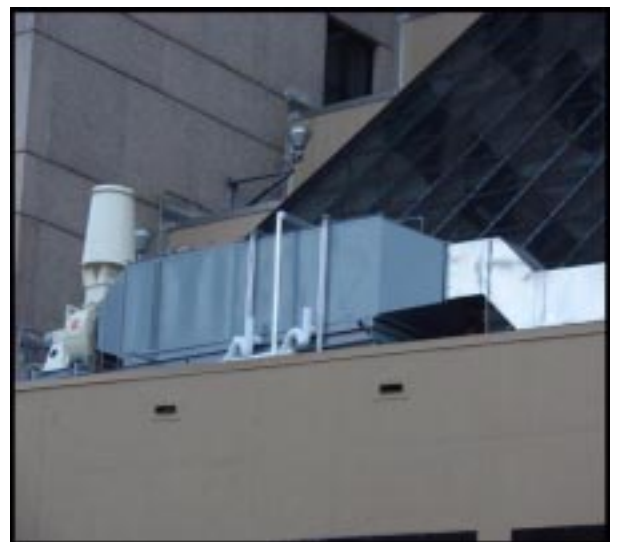
12,000 cfm K-Pack Rooftop Installation
